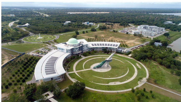
Figure 1. Universiti Malaysia Al-Sultan Abdullah (UMPSA) in Pekan, Pahang, Malaysia
