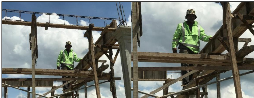
Figure 10. Construction Workers Work While Unzipping The Front To Get Natural Ventilation
